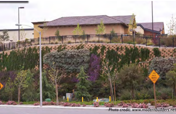
The VERDURA Living Retaining Wall system is a fully plantable block wall that is Caltrans approved.
