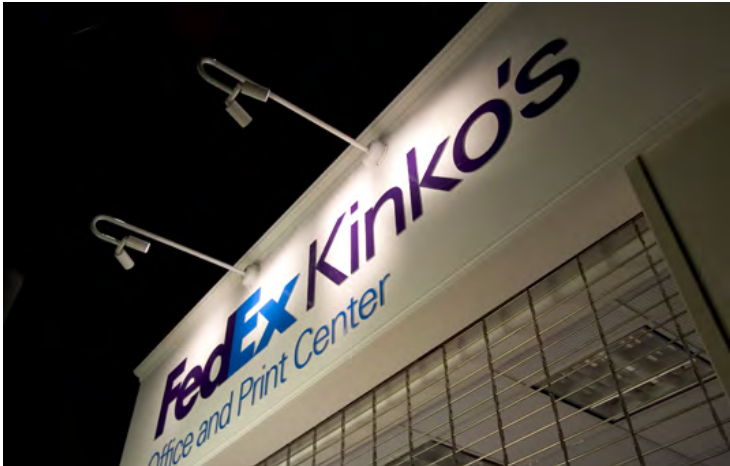
Sign lighting that faces down to reduce light pollution: B-K Lighting Twin SignStar Style A
