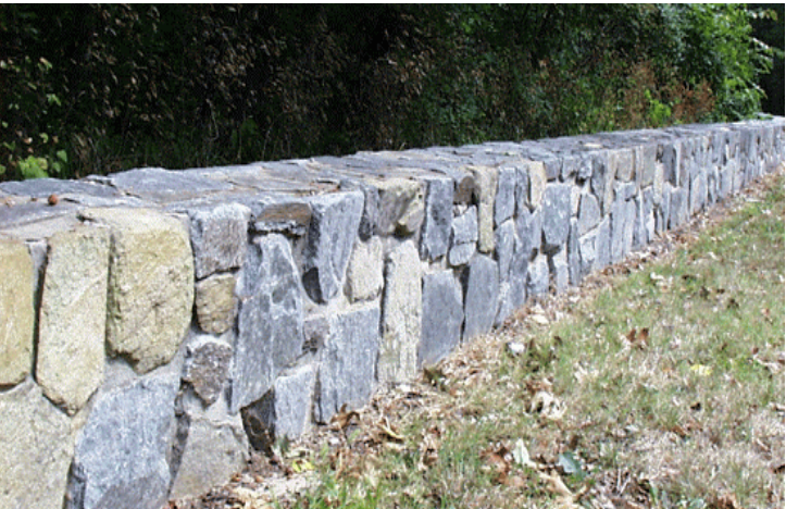
A Stone Masonry Guardwall consists of concrete faced with natural stone. Above: Caltrans guardwall in San Luis Obispo.
