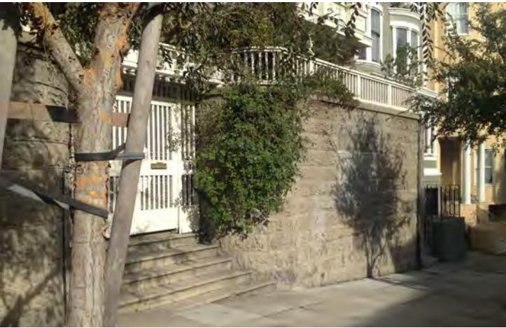
A structural, reinforced concrete retaining wall is covered by a sculptured veneer treatment and further softened with a railing and foliage.
